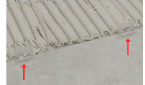
Image 32: Leveling spacer
