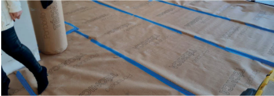
Image 46: Applied floor protector
