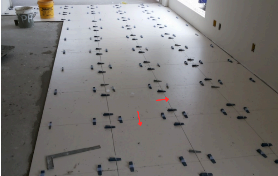
Image 42: Wedges in the same row must be inserted in the same direction.
