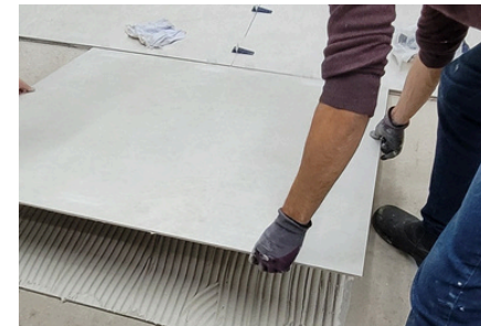
Image 33: Execution of dragging on the piece.
