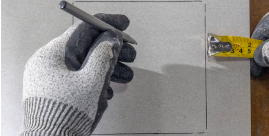
Image 79: Draw the cut to be made on the piece.
